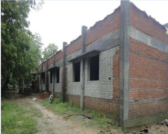
Saraswati Girls Hostel (Under Construction)
