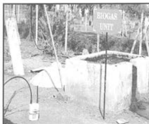
Fig.4. Two cubic meter modified Janta biogas plant
