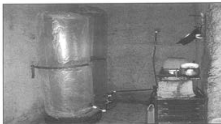
Fig. 1.12 : Gas Holder and Gas Storage Reservoir
