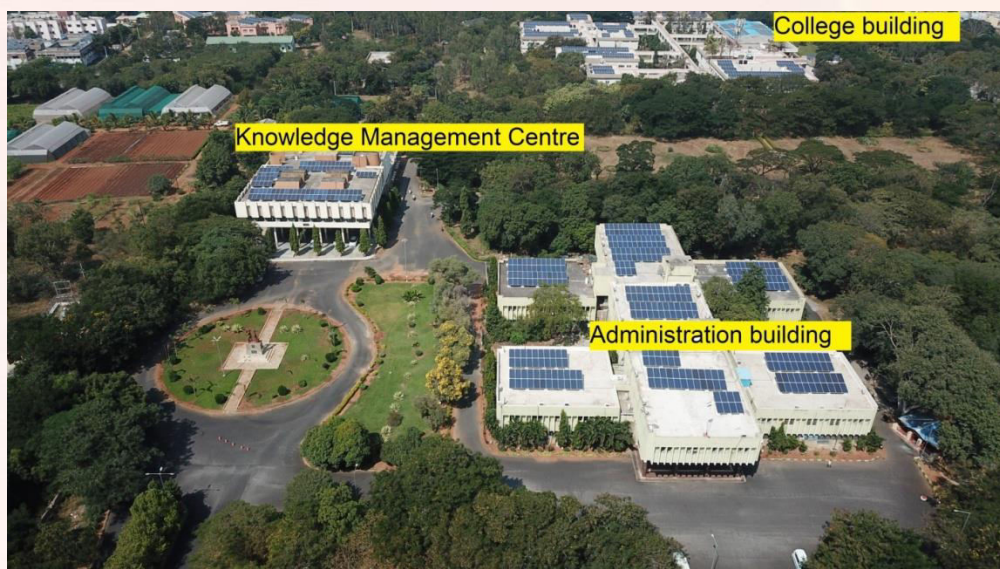
Solar panels at Professor Jayashankar Telangana State Agricultural University (PJ TSAU), Hyderabad
