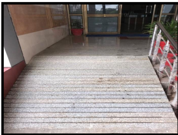
Barrier free access for the physically challenged
